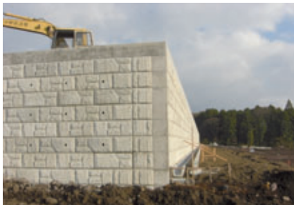
Fig. 2: Golcon Block with designed surface
