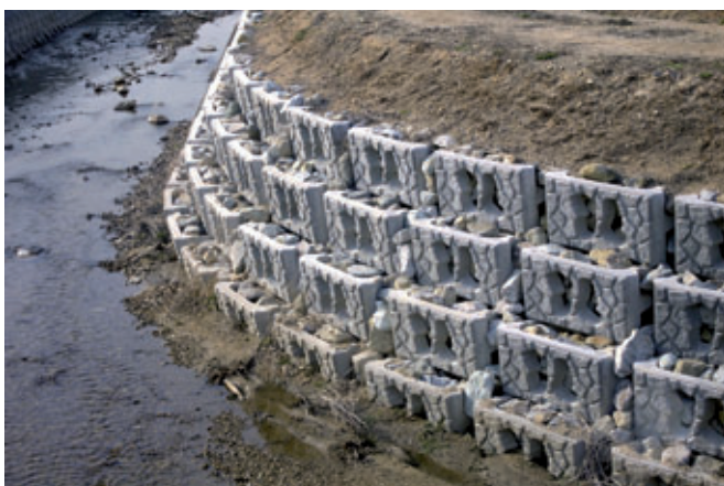
Fig. 1a, 1b: Hollow concrete blocks - mainly used for river revetment
