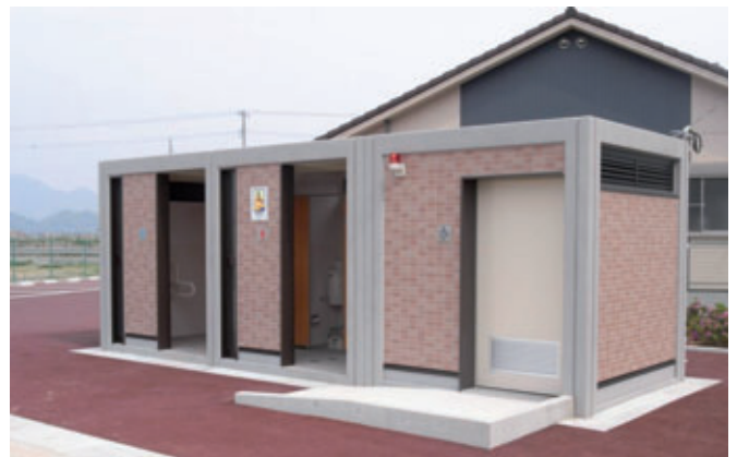
Fig. 2: Public lavatory in a park
