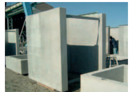
Precast elevator shaft subassemblies transported to the construction site.
