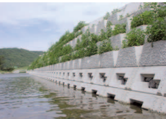
Fig. 2a, b, c: Block examples which enhance the function for both revetment and eco-friendly.
