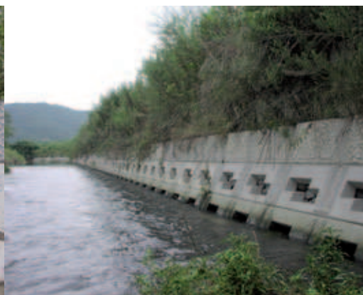
Fig. 2a, b, c: Block examples which enhance the function for both revetment and eco-friendly.
