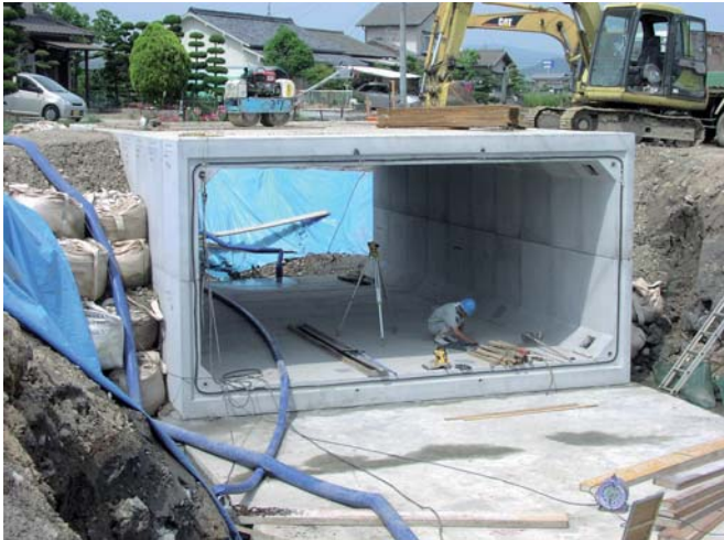
Fig. 1,2: Box culverts at construction site
