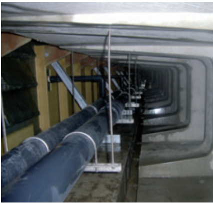
Fig. 6: Swimming pool construction
